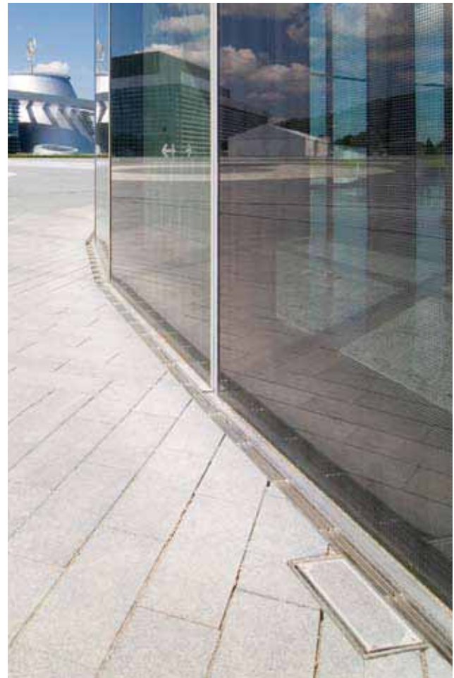
The facade is drained via a channel with a longitudinal bar grating and removable side wall. Special inspection boxes provide access to the channel.
